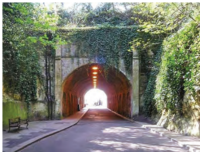
View into Reigate Tunnel from the north
